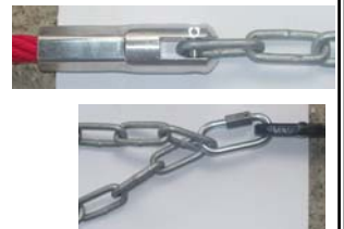
CHAIN USED FOR ATTACHMENT OF NET IN LOOSEFILL. PULL TIGHT & CUT OFF THE EXCESS
